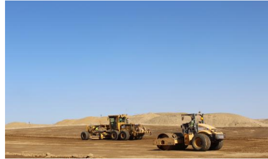
DG II Enabling works - DGCL
