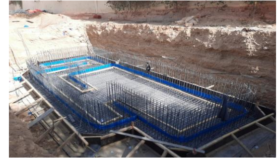
Constructing of MISK City Infra structure Package - MISK
