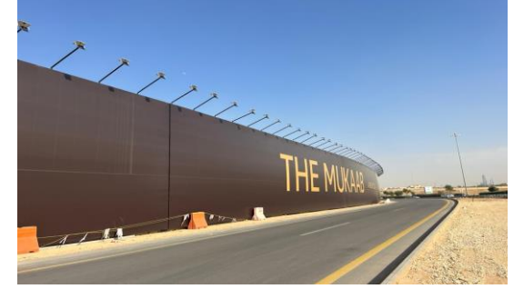
Site Hoarding Works, & chain link fencing startup site - NMDC
